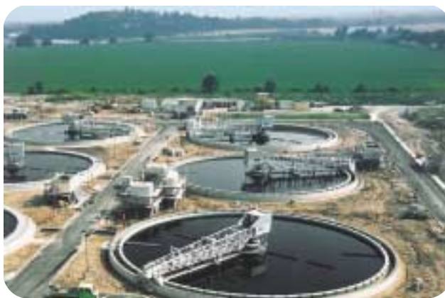
At waste water treatment plants
