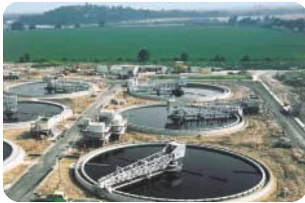
At waste water treatment plants
